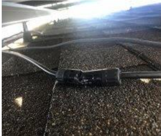
Defective cable replacement
