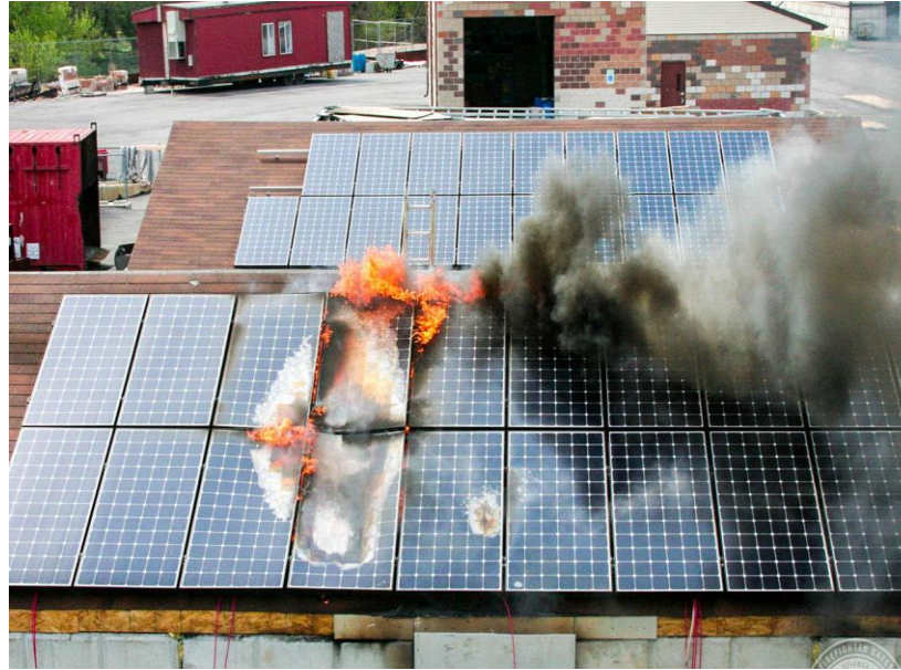
Fire due to PV panel
